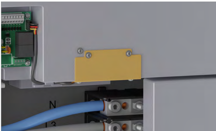
Position of internal fan 1
